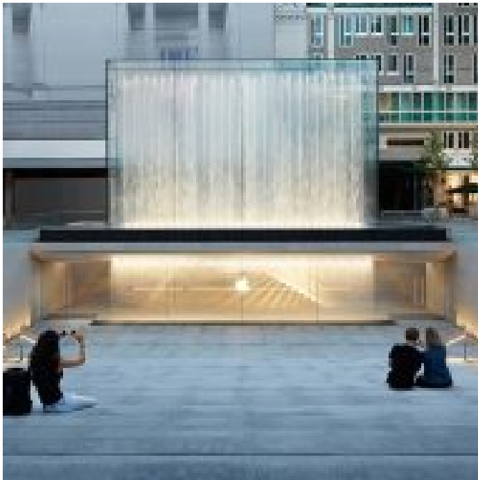
Fountains jet water over entrance to Foster + Partners' sunken Apple store in Milan
